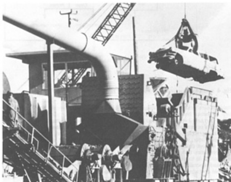
Fig. 3 Junked automobile being fed into a shredder. Courtesy of the Institute of Scrap Recycling Industries, Inc.
