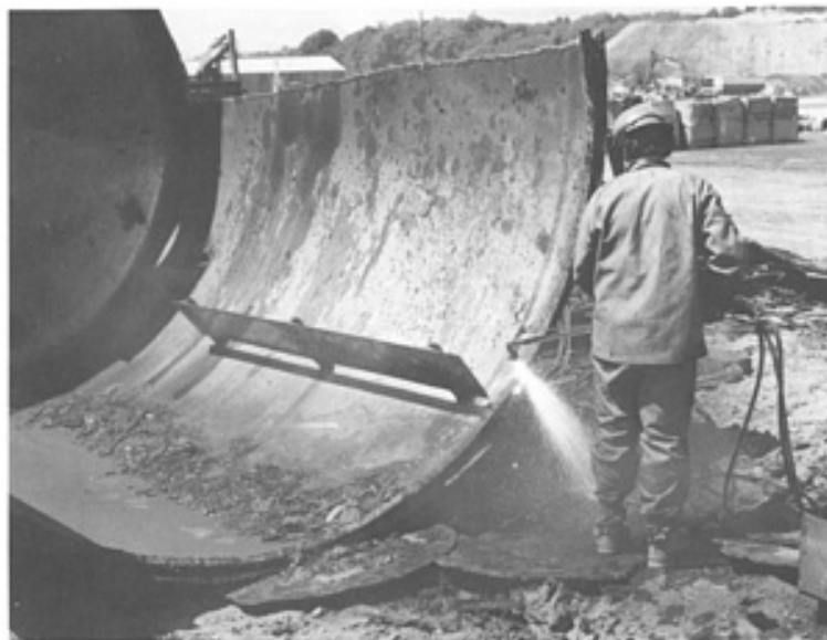
Fig. 2 Large tank being cut down to size with a torch. Courtesy of the Institute of Scrap Recycling Industries, Inc.
